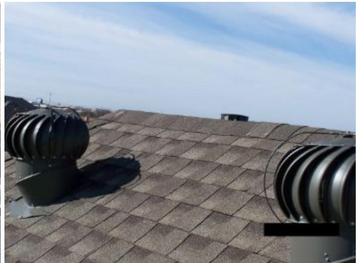
Wind Turbine Vents: 4 present and operating at time of inspection
