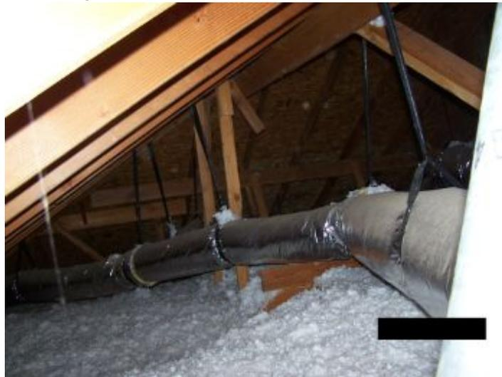
Blown in Fiberglass insulation: approximate depth 8-10"
