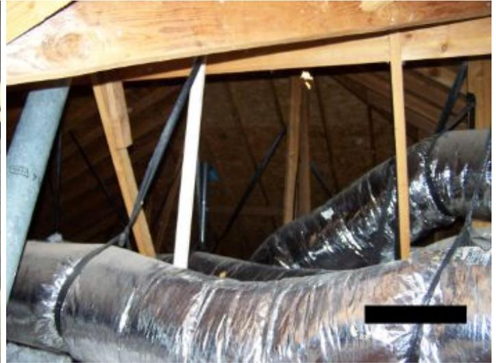
Air Duct Strapping in place
