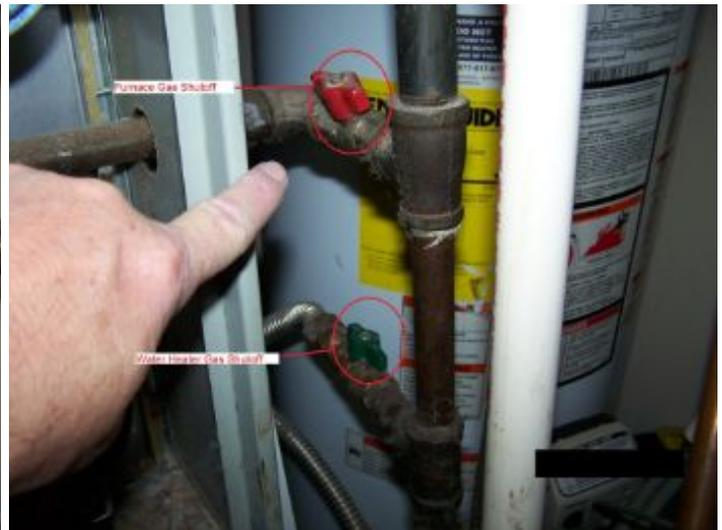
Gas Cutoffs for Furnace and water heater located adjacent to units
