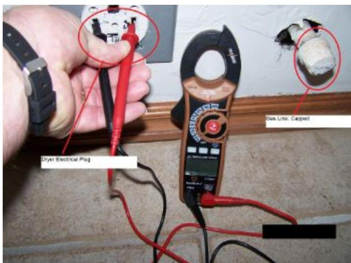
Power to dryer verified: note gas line for dryer present but capped.
